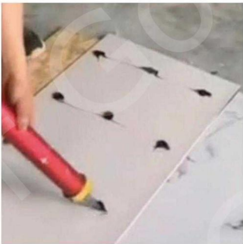
·Step 3 Apply nail free gule to the back
