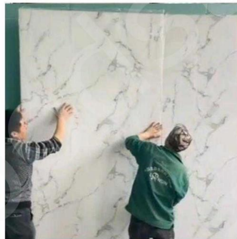
·Step 4 Paste it on the wall.
